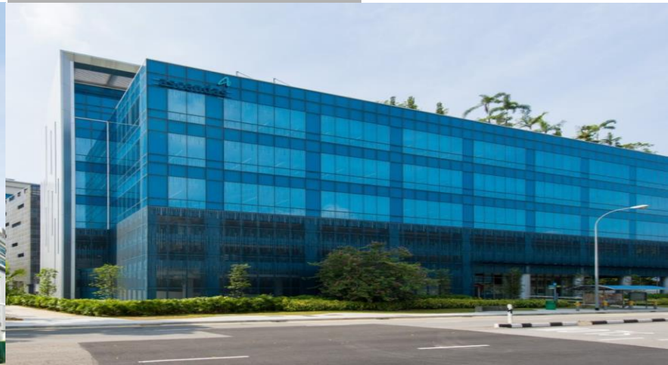
DNV GL Technology Centre
