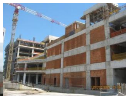
Mar 09: Construction in progress
