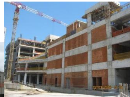
Mar 09: Construction in progress
