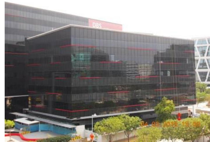
Completed Ph 2 block at DBS Asia Hub
