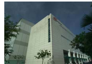
IDS Logistics Corp HQ
