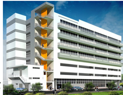
Techplace II upon completion of asset enhancement
