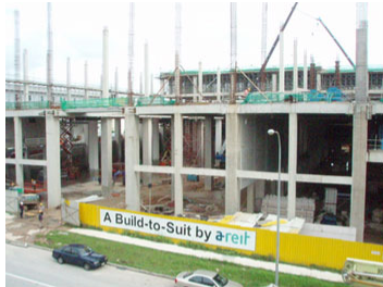
Dec 2007 – construction under way
