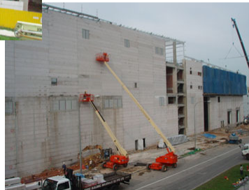
Mar 2008 – construction in progress
