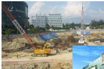
Mar 08: Construction of Phase 1 in progress
