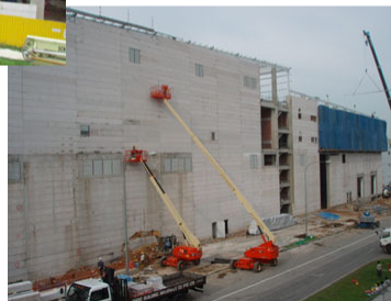
Mar 2008 – construction in progress
