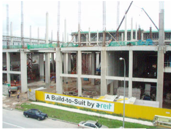
Dec 2007 – construction under way
