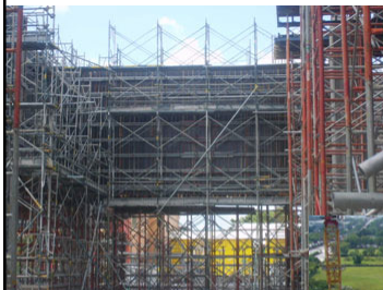
Dec 07 – Construction on schedule
