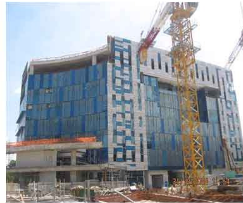
Dec 08: Construction of Phase 1 building on schedule
