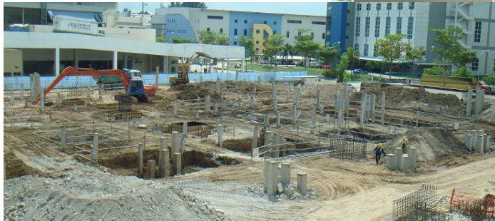
Dec 2008 – construction in progress
