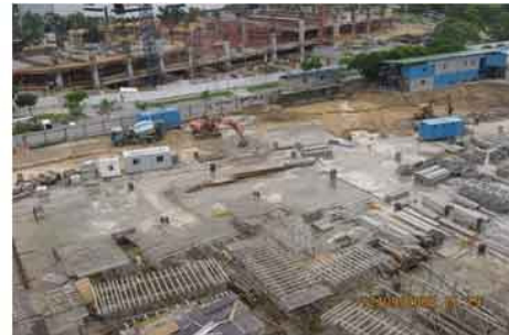
Sept 08: Commenced construction of MTB Building
