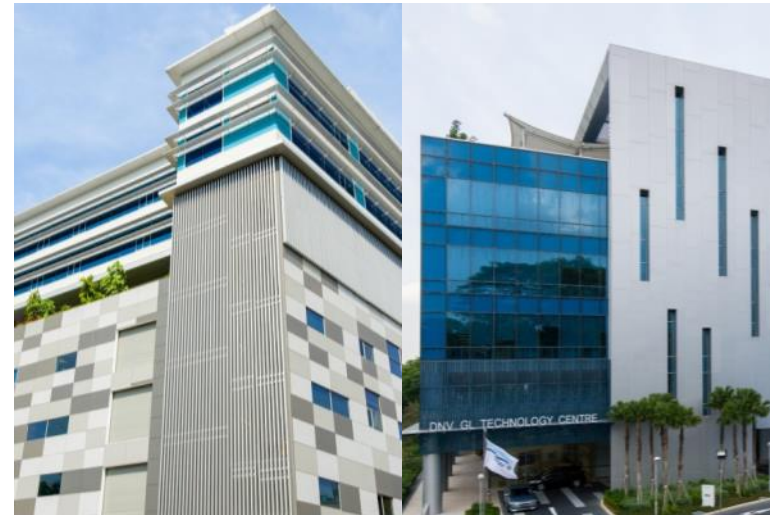
LHS: DSO National Laboratories, RHS: DNV GL Technology Centre
